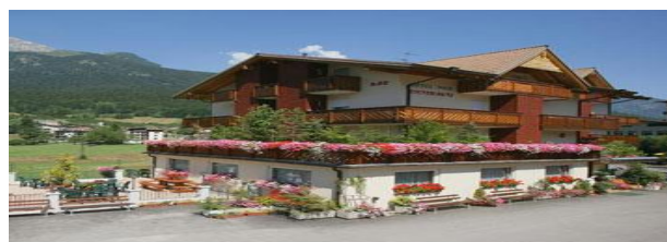
Hotel Pier Andalo – Hotel Zodiaco
